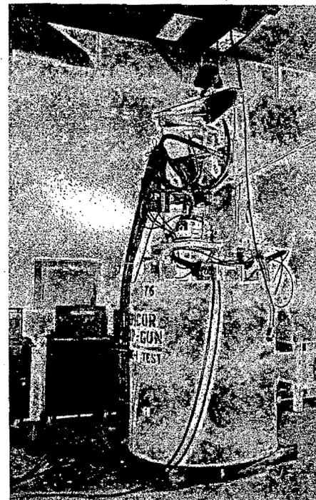
Figure 21 Prototype gas sampler installed on EPICOR II liner.
