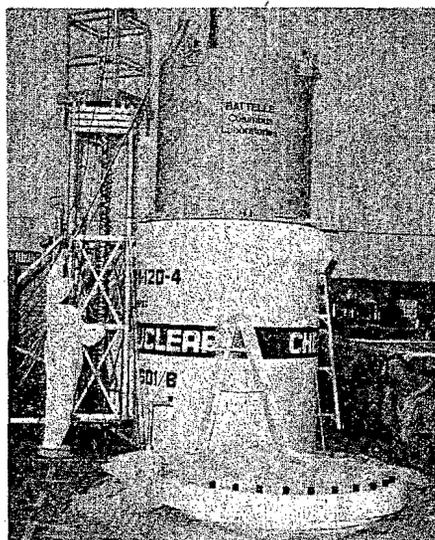
*Figure 15* BCL transfer and storage device atop the PF-16 shipping cask.
