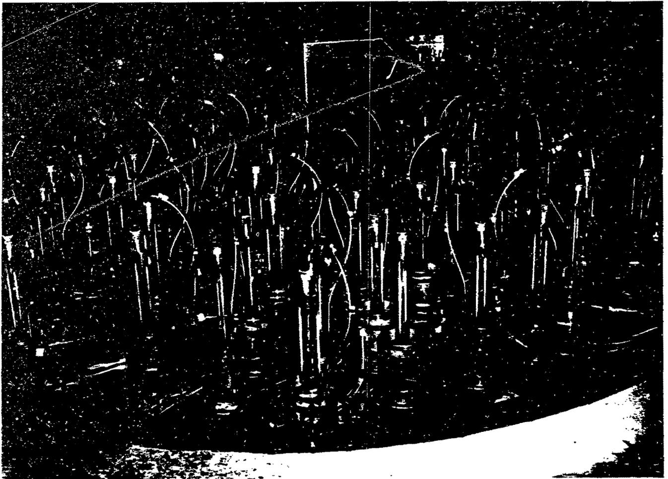
Accumulation of boron crystals is evident around the base of the incore instrumentation seal table. Corrosion is visible on the exposed metal surfaces.
